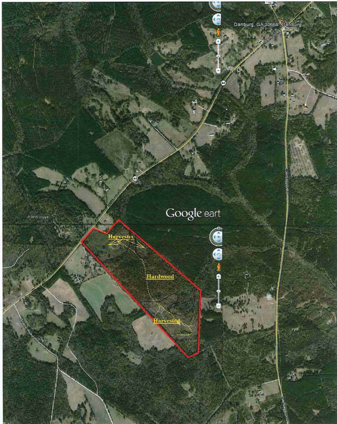
Aerial Photograph Rivers Tract 108.33 acres Wilkes County, Georgia Scale: 1" = 1,200' Date: December 16, 2015 James I. Alfrend Consulting Foresters, LLC
